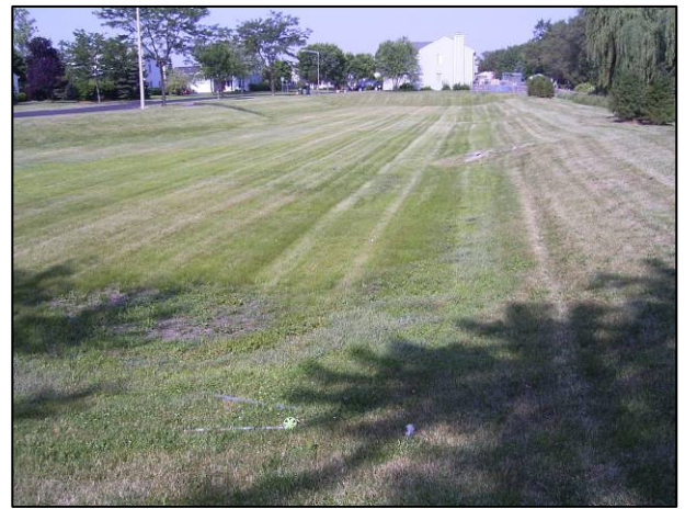
Figure 5.30: Typical dry bottom basin
