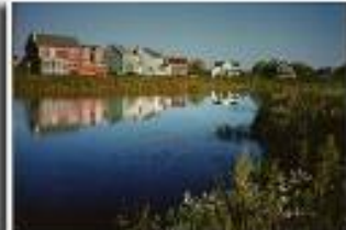
Regional Detention Basin with Constructed Wetland and Sediment
