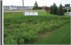
2. Bio-Filter Infiltration Basin
