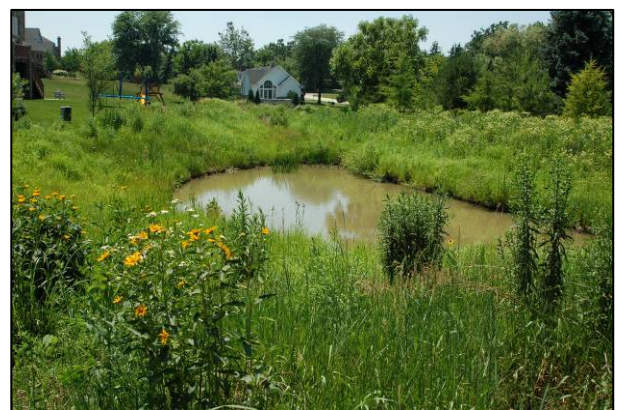
Figure 5.32: Naturalized Detention Basin
