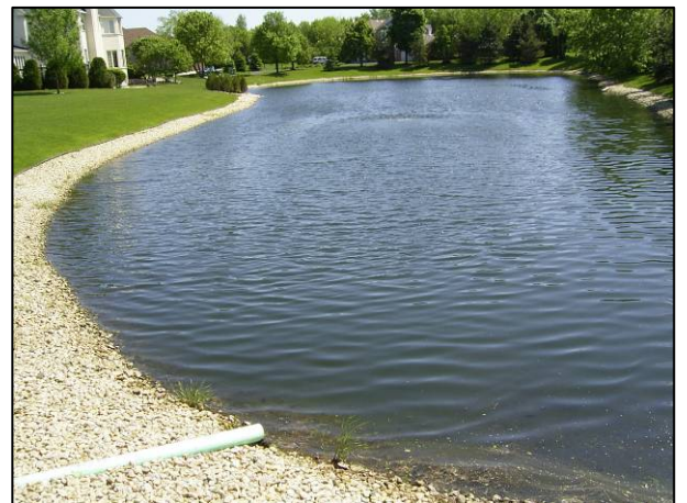
Figure 5.31: Typical wet bottom basin
